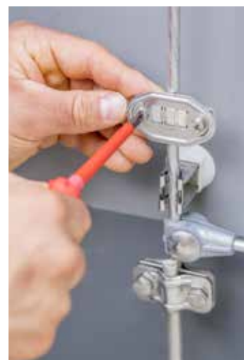
Fourth step: Fix the marked number plate at the down conductor.
